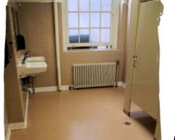
Key Broadcast Quartz Flooring sets the standard for decorative resinous flooring systems. These systems are installed between <sup>1</sup>/<sub>16</sub> and <sup>1</sup>/<sub>4</sub> inch thickness and are available in a variety of standard color blends. With or without the integral cove base, they provide a non-porous, seamless finish that resists deterioration by water, food and chemical spills and is resistant to bacterial growth. The installed system can be textured or smooth as desired.
